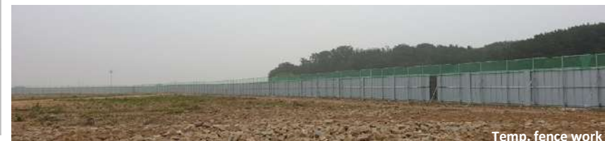
Temp. fence work
